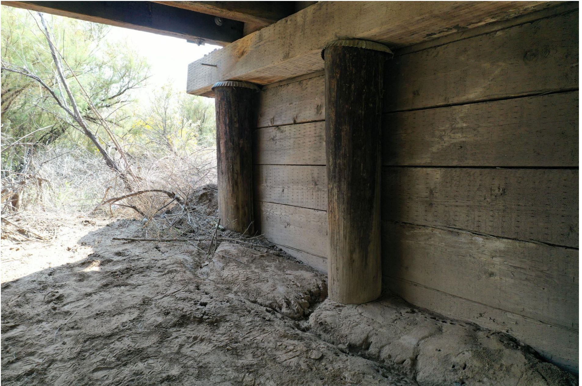
WATER STAINING ON EXISTING ABUTMENT STRUCTURE O-19-D FIGURE 2
